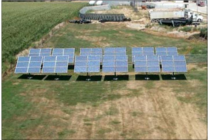
*Twelve, grid-tied solar arrays (six modules per array) are now producing power at the FEC Solar Garden. Energy production can be monitored online. Visit [www.feckalona.com](http://www.feckalona.com) and click "View Production Data" in the left column.*
